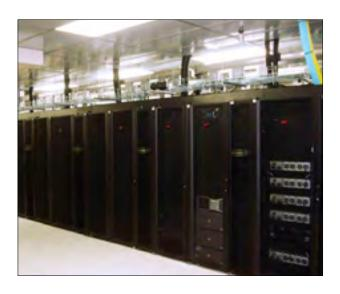
All power within the data center is distributed via overhead buss from the PDU's. The completed second phase houses 21 racks of IT equipment.
